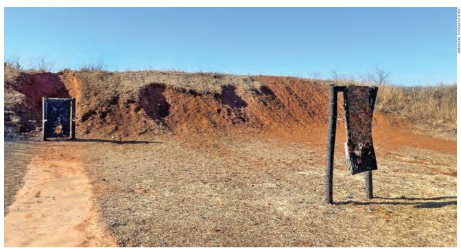
Apparent in this photo is the degradation of the backstop berm at Cherokee WMA's shooting range. Berm replacement is part of the renovation process for existing shooting ranges.
