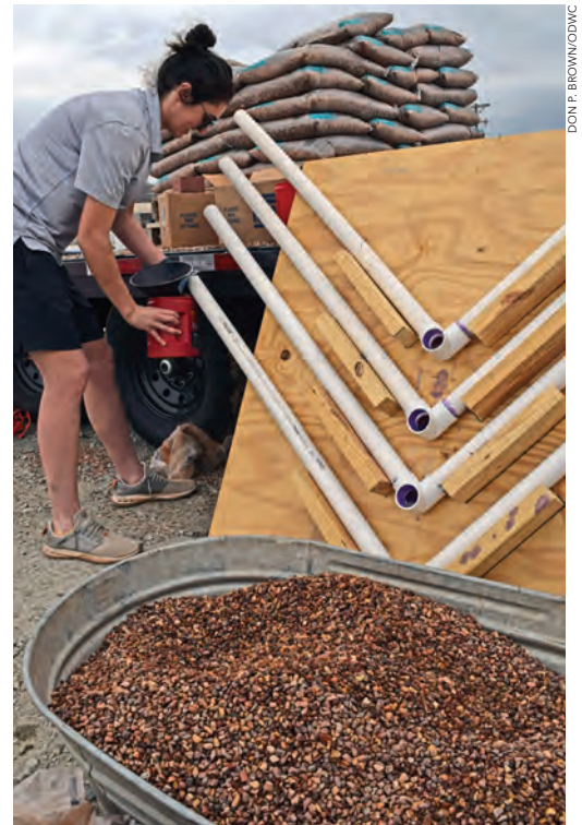
An ODWC Fisheries staffer fills fish habitat cube frames with gravel to hold them in place on the lakebed.
