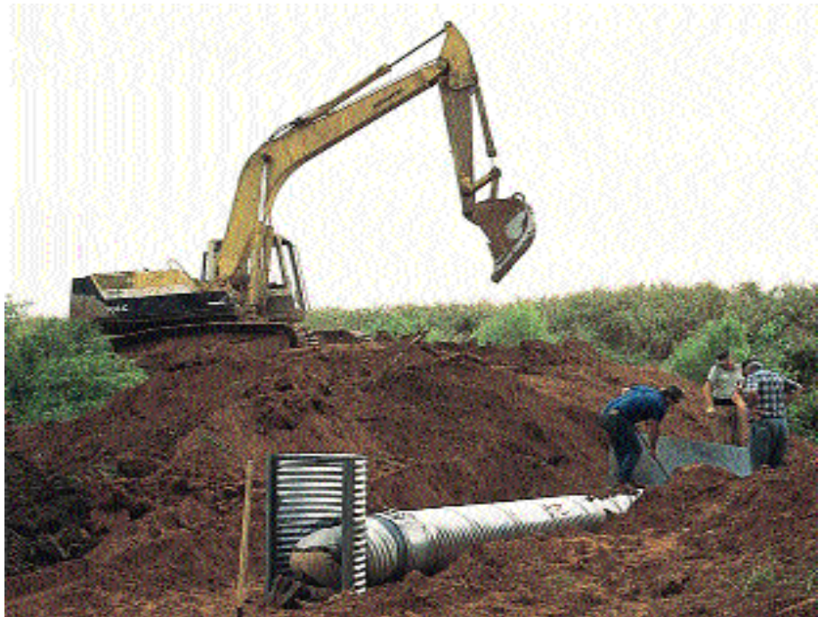
Landowners may receive technical assistance for wetland restoration projects, including water control structures for wetland management such as the one seen above. These projects will attract a variety of wildlife for a landowners enjoyment.
